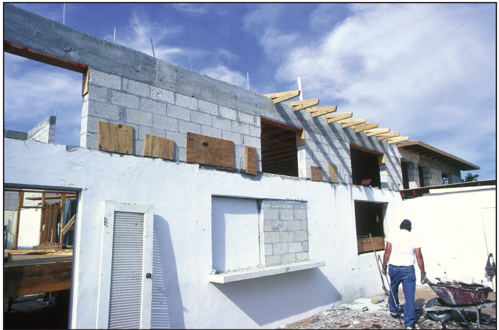
Figure 67 The extended first-story walls.
